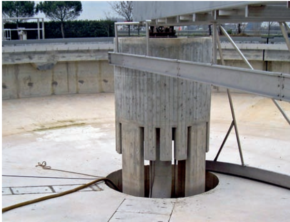
Photo 3. Sedimentation tank (empty)
